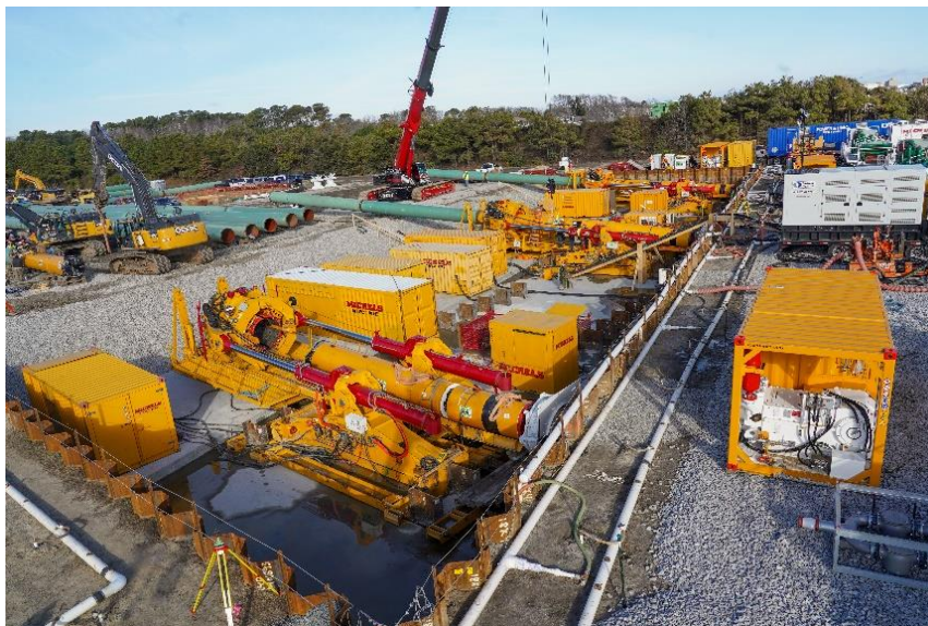
Figure 8. 3x Direct Pipe 42 inch equipment with jet pump in operation on Coastal Virginia Offshore Wind Project, for 9 export cable landfall drives (Michels Trenchless Inc., USA)
