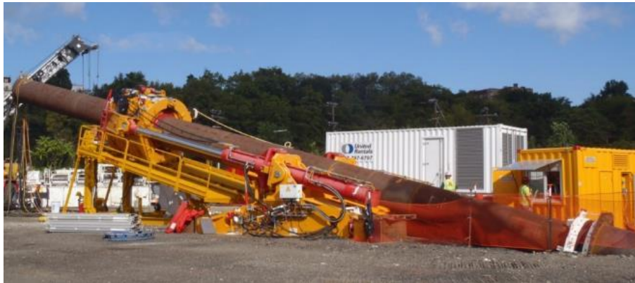
Figure 11. Retractable Direct Pipe MTBM used for New Jersey Expansion Project, USA, for 48" HDD casing of 85m length
